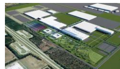
HL-GA Battery Project Georgia, USA
