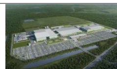
S-JV Battery Cell Project Georgia, USA
