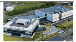
Takasago Thermal Engineering Innovation Center, Japan
